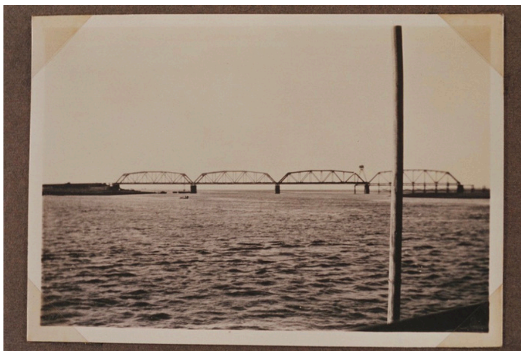
Fig. 5 White Nile bridge between Khartoum and Omdurman during construction. From the papers of Mabel Elsie and Gertrude Lucy Wolff within the Sudan Archive, Durham University Library and Collections (SAD.743/2/23)
